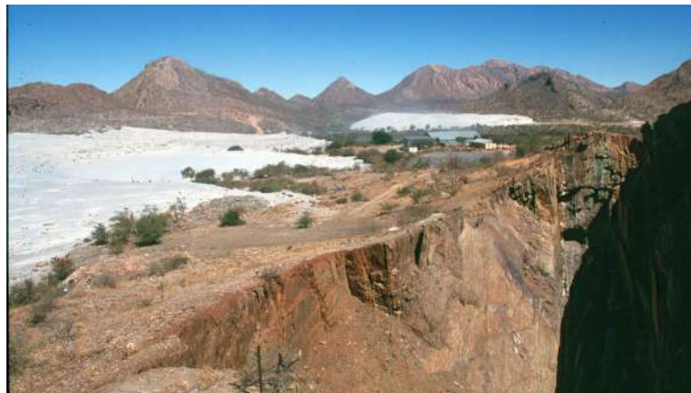
An abandoned mine from pre-independence. The importance of properly implementing the Environmental Management Act to prevent damaging consequences cannot be overstated.
